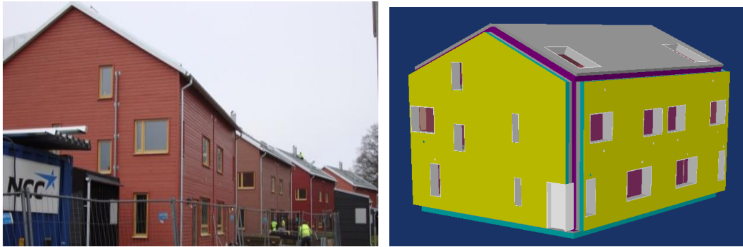
Figure 9. Left: Four identical two-family houses in Stockholm; Right: simulation model frame of the houses in the IDA ICE 4 software
